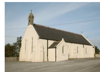
St Colman's Derrinacantha Church
